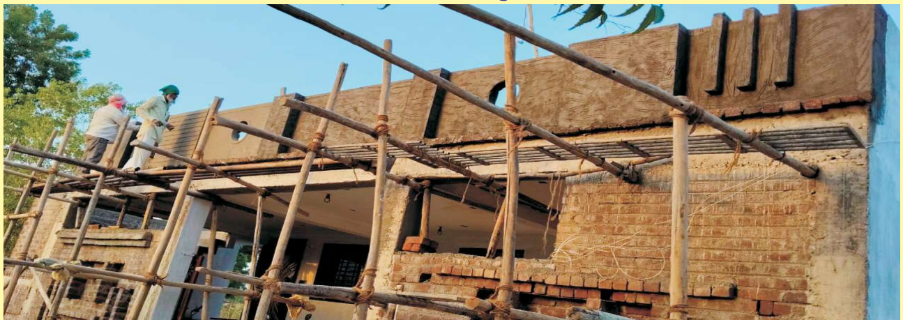
One of our under construction church buildings
